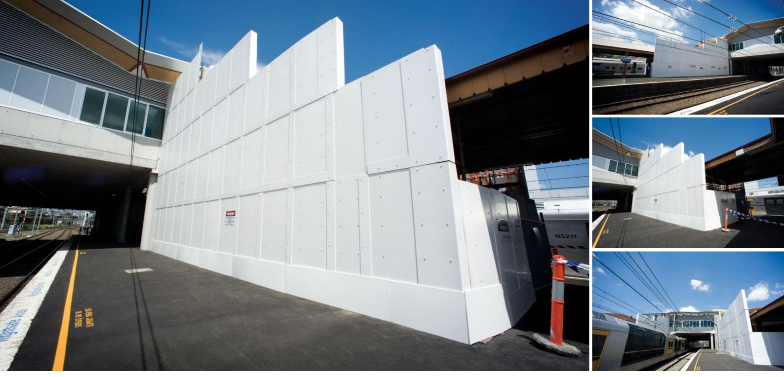
In total, Synergy Scaffolding supplied approximately 300 tonnes of scaffolding to the Sydenham Station upgrade, including access ladders with tie-down hatches. Every scaffold was a separate unit, with no connection possible, and spread over six platforms.
