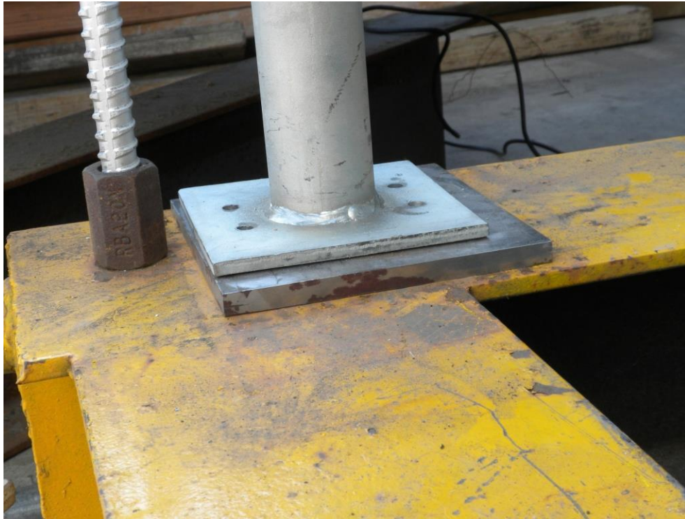
Photo C: Slop base for test
